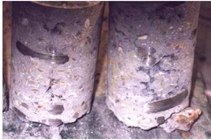
Permanent sprayed concrete samples containing 12mm diameter steel reinforcement
