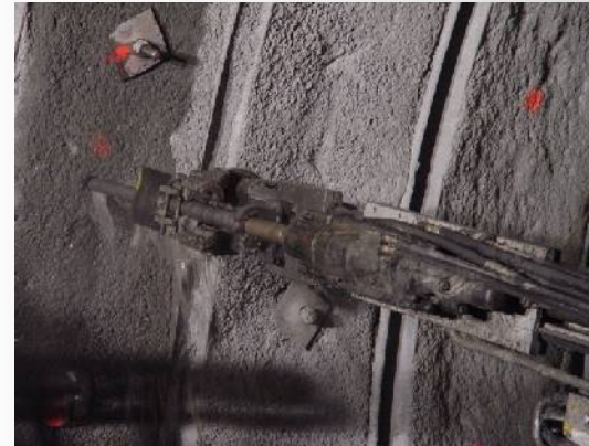
Selfdrilling friction bolt AT-Power set
