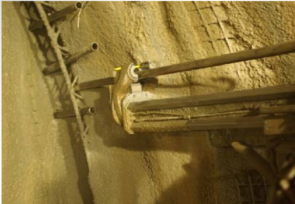
Short forpoling System AT-Self Drilling-Tube Spile
