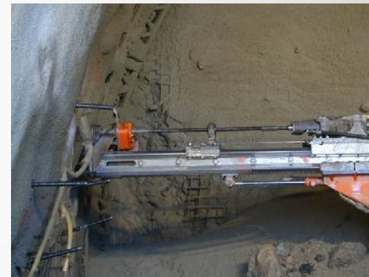
Self-drilling injection bolts IBO / IBI bolts
