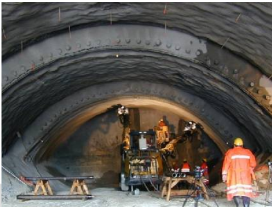
Long forpoling System AT-Casing Systems
