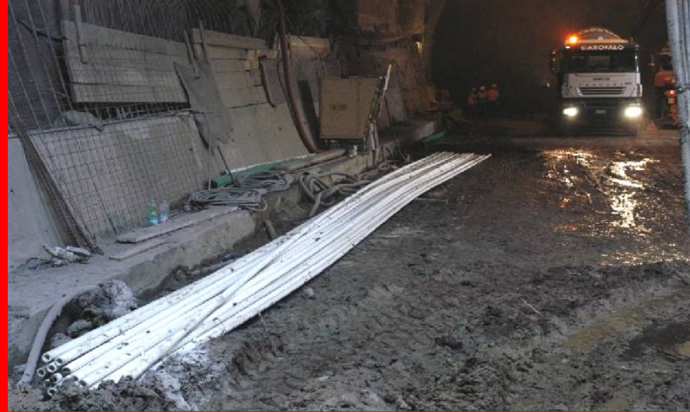
PHASE 2: Positioning pipes
